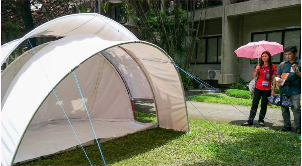
The Kuhol Tent Model (snail in English) uses easy-to-find materials assembled and shaped to keep the interior dry and cool in harsh weather conditions. It has two sections: an exposed floor anteroom that can remain open to allow air through, and an inner sleeping quarter.
