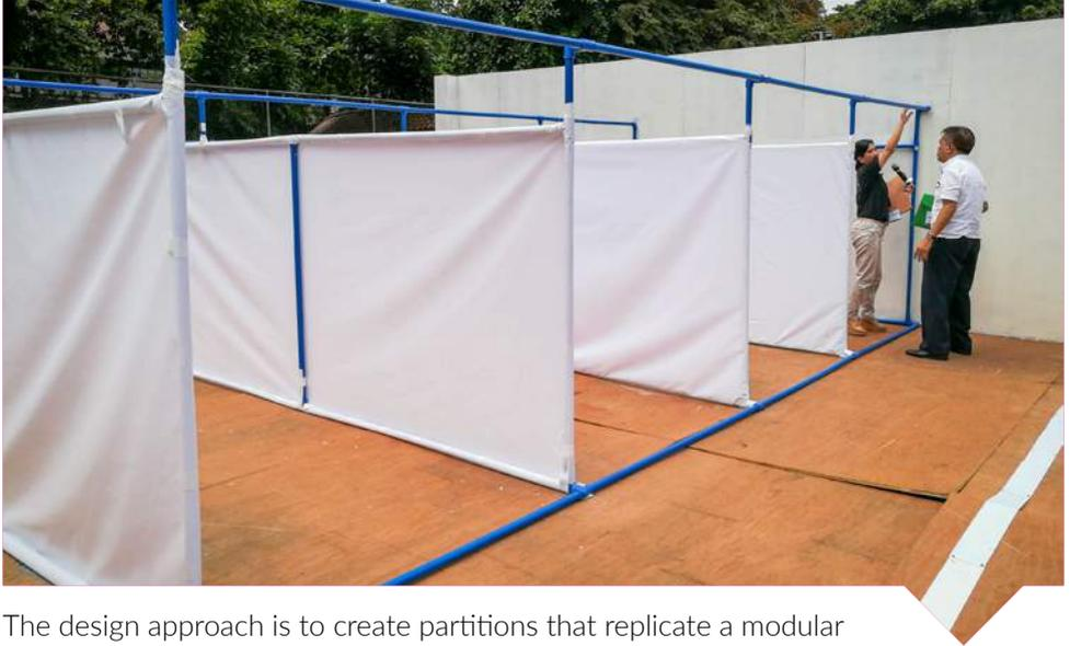
The design approach is to create partitions that replicate a modular system that can be used individually, or as components of a bigger ATS unit. The Temporary Classroom Partition (TCP) can be adapted depending on the spatial and social requirements of the evacuees. It addresses common issues encountered in classrooms being used as evacuation during disasters.
