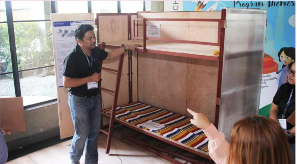
This temporary shelter model is a scalable planning system of ready-made compact modules comprised of built-in hinged wall and door panels that unfold and join together with other modules to form private lockable units with beds.
