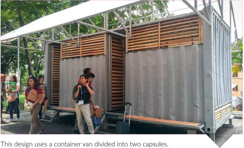
This design uses a container van divided into two capsules. The opening on its long side is fitted with lightweight metal panels that allows for operability. When opened, this can serve as the front roof for the lanai that is accessible by a ladder. The dividing panel uses recycled pallet wood slotted into metal frames, the same one which can be fitted with a shelving system. However, if there is a need to utilize the full length of the van, the partition can be removed.
